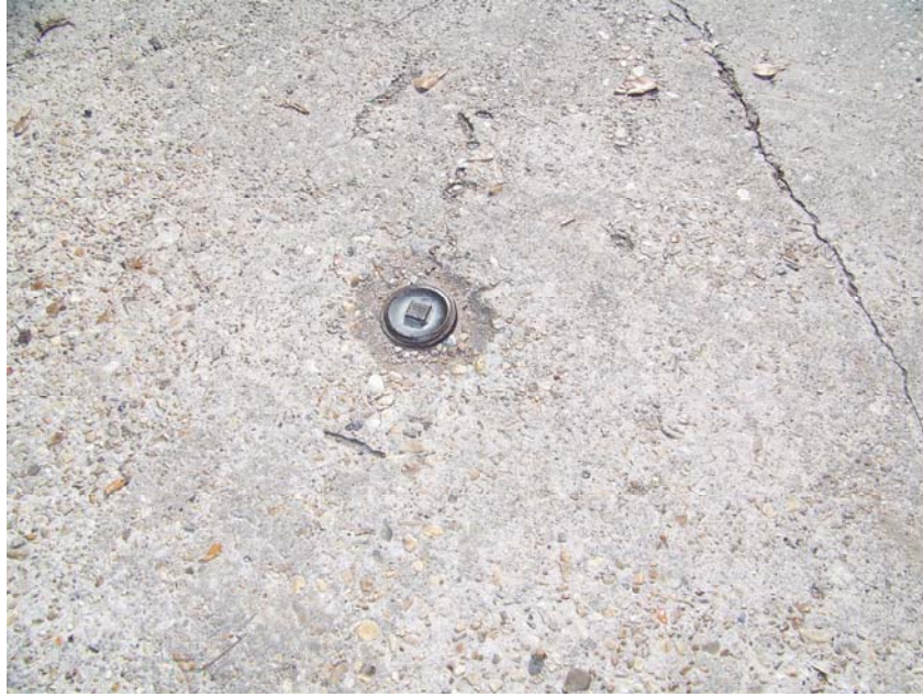
Photograph 9. Possible Fill Port at 453 East Main
