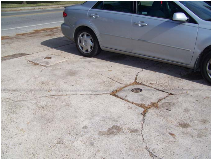
Photograph 6. Fill Ports at Former Twin Gulf Service Center
