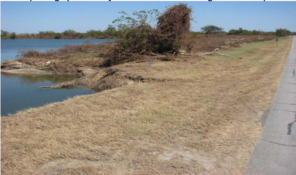
Photograph 4.3.4 Easterly ground level view of Trosclair Road sand pits in Cameron Parish following Hurricane Ike. (Photograph courtesy of CMD Permits and Mitigation Section).
