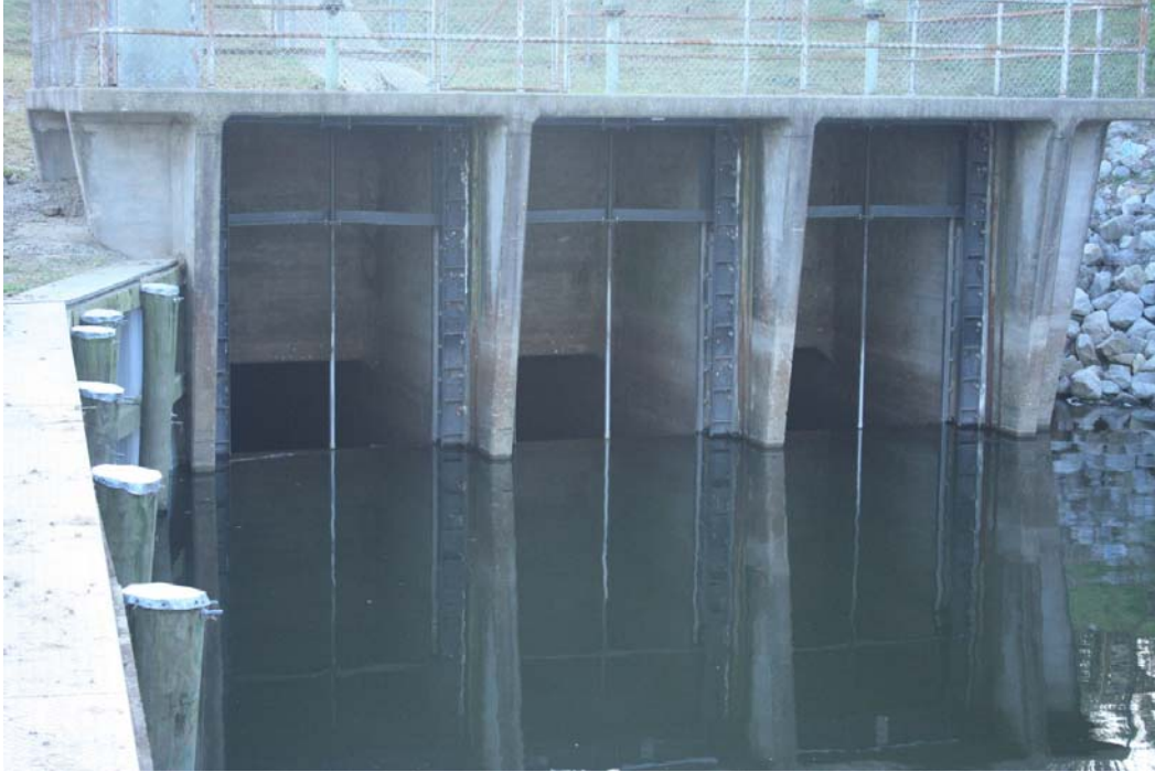
Figure 1. False River Control Structure gates. False River is behind the photographer and the Louisiana Highway 1 and box culverts are behind these gates.
