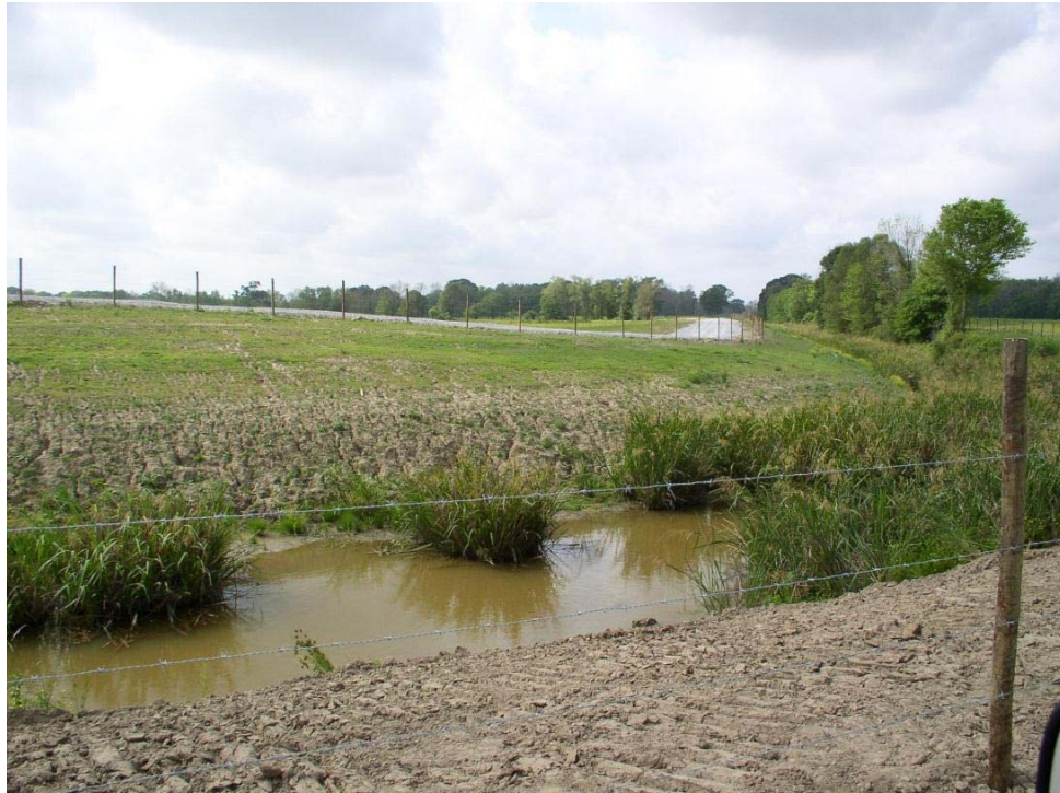
Figure 4-17. Post-construction Photograph of the M-1 Canal Showing the Fences and the Bank Dressing Performed by NRCS (courtesy of NRCS, New Roads, Louisiana)
