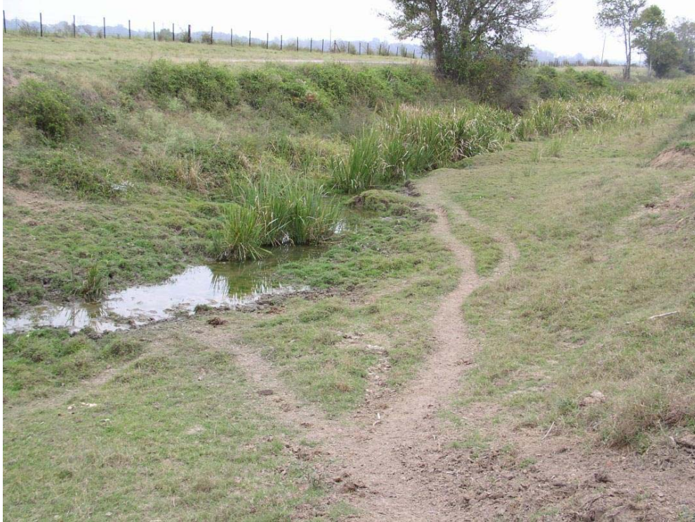
Figure 4-13. M-1 Canal before EQIP Project Showing Erosion Created by Cattle (courtesy of NRCS, New Roads, Louisiana)
