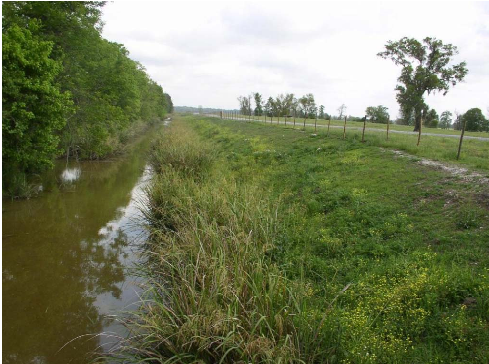
Figure 4-18. Post-construction photograph of the M-1 Canal Showing the Fences and the Bank Dressing Performed by NRCS (courtesy of NRCS, New Roads, Louisiana)
