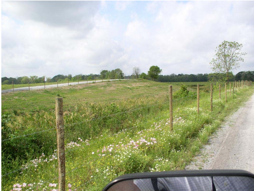
Figure 4-15. Post-construction Photograph of the M-1 Canal Showing the Fences and the Bank Dressing Performed by NRCS (courtesy of NRCS, New Roads, Louisiana)
