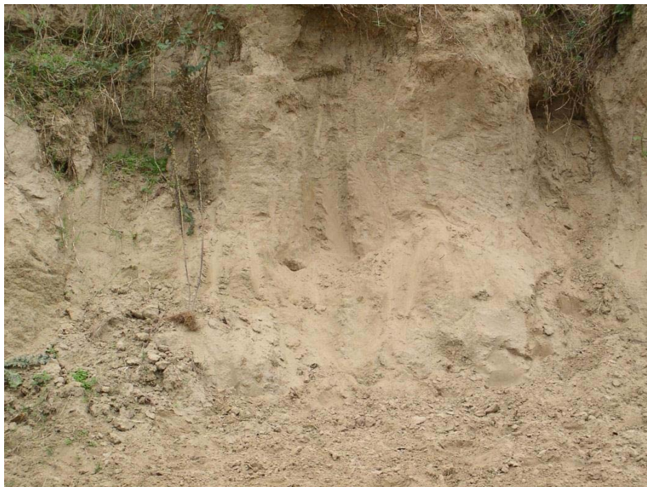
Figure 4-12. M-1 Canal Before EQIP Project Showing Erosion Created by Cattle (courtesy of NRCS, New Roads, Louisiana)
