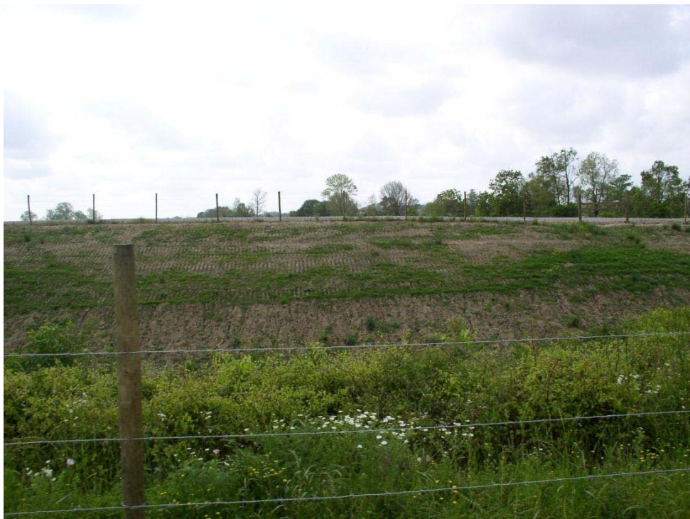
Figure 4-16. Post-construction Photograph of the M-1 Canal Showing the Fences and the Bank Dressing Performed by NRCS (courtesy of NRCS, New Roads, Louisiana)
