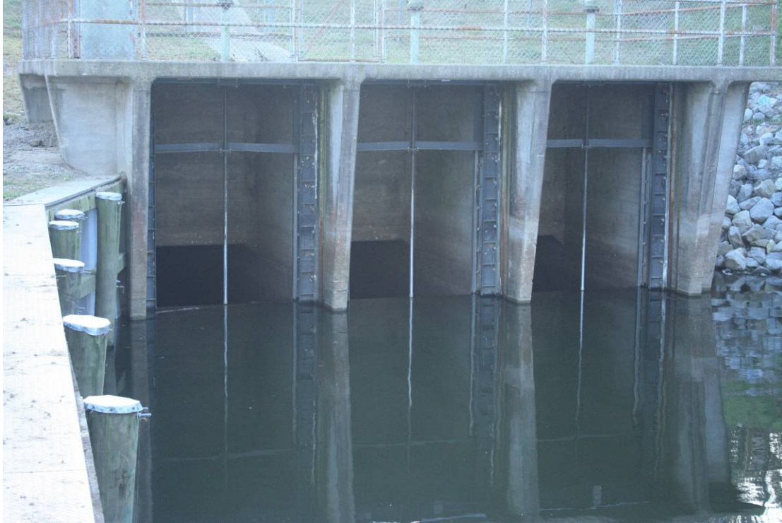
Figure 4-4. False River Control Structure Gates. False River is Behind the Photographer and LA Hwy 1 and Box Culverts are Behind These Gates
