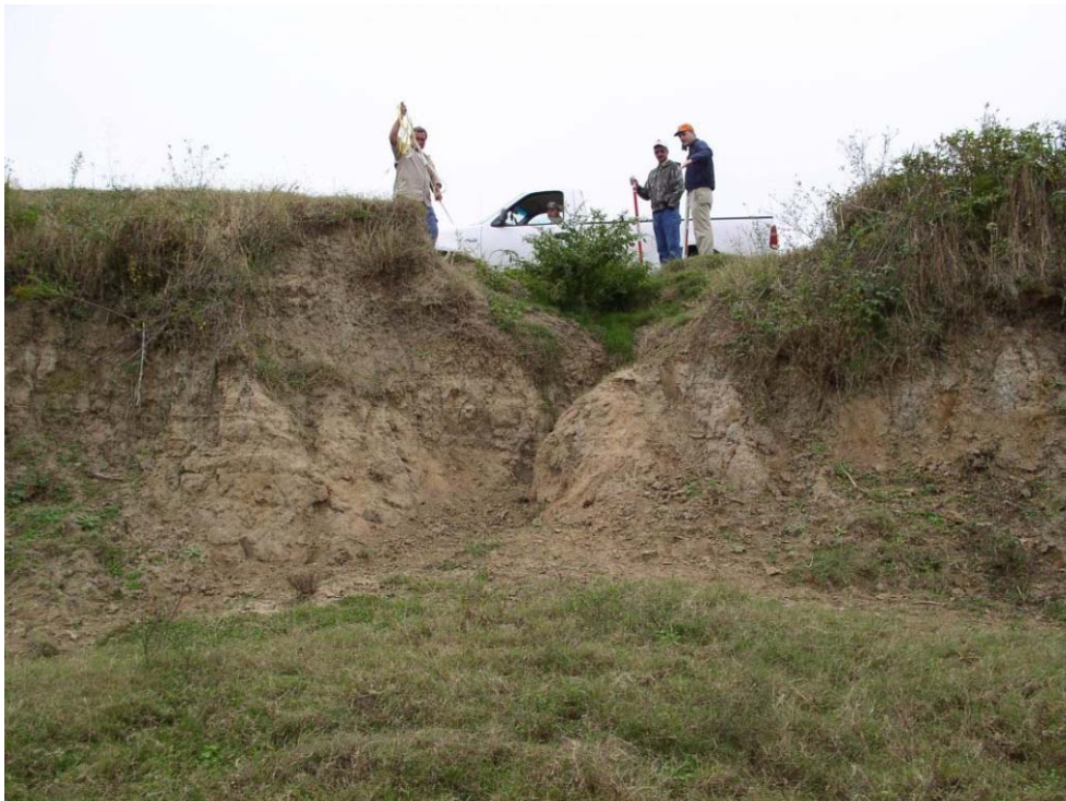
Figure 4-14. M-1 Canal before EQIP Project Showing Erosion Created by Cattle (courtesy of NRCS, New Roads, Louisiana)
